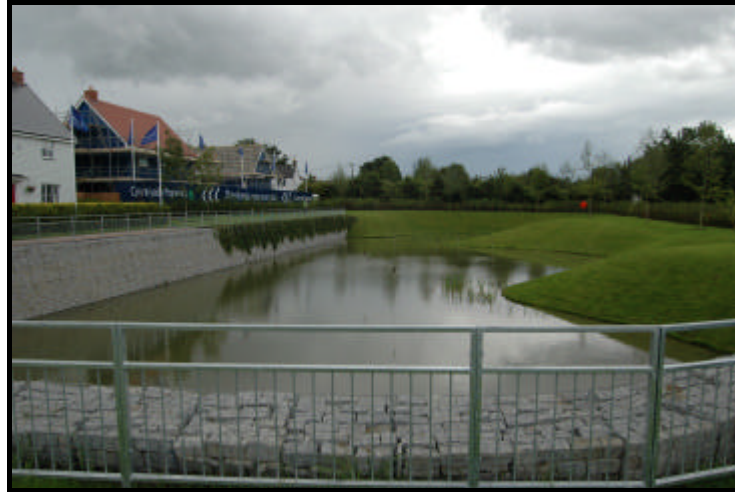
Figure 8.1: Balancing pond at Prior's Green Takeley.
