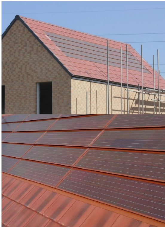
Integrated photovoltaic clay-type roof tile (source: Romag)
