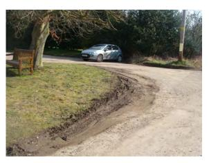
Picture 1.24 Small green near church whose edges are badly eroded by vehicles
