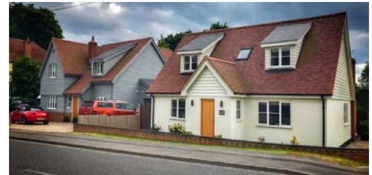
Photo 27. Recent (2016) Housing development on High Street (south side); to left- house new build and right - reconstruction and extension
