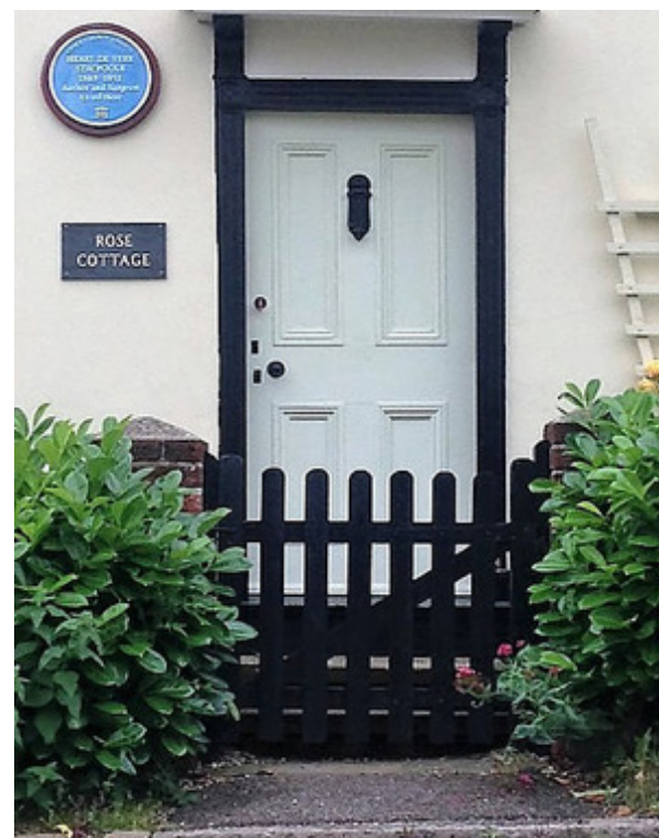
Photo 9. View of House Facade at Church End
