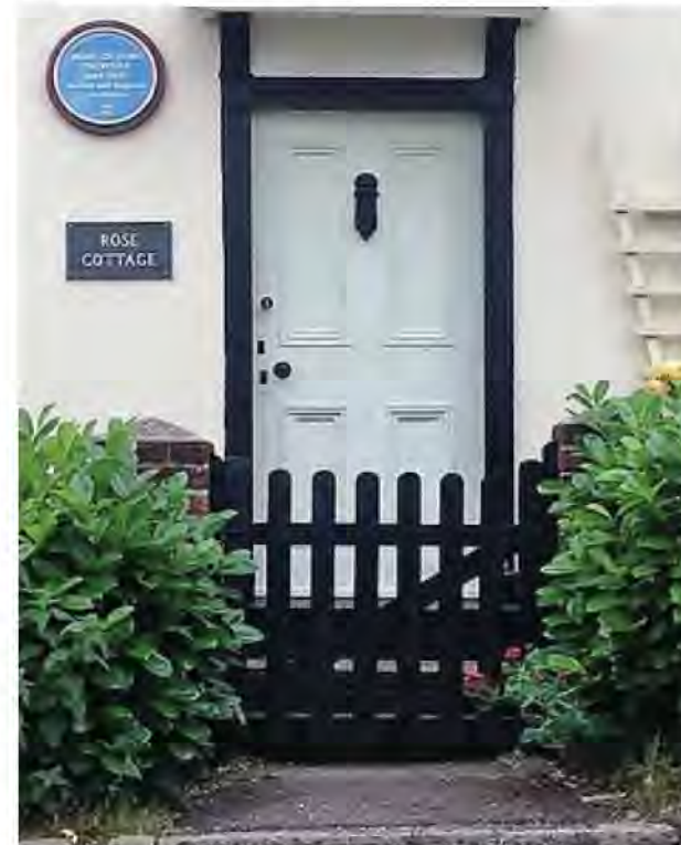
Photo 9. View of House Facade at Church End
