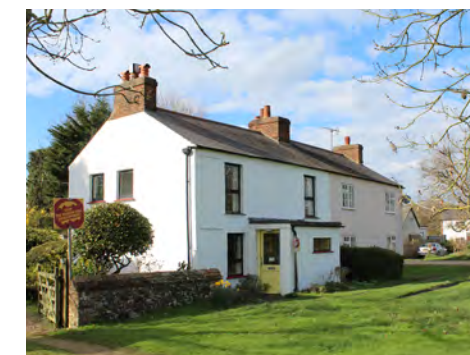
Figure 29 South and Smiths Cottage
