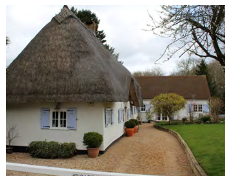
Figure 22 Hollow Elm Cottage
