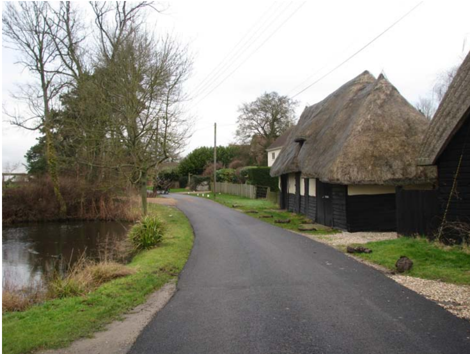
Farm complex bisected by lane (lane 102)
