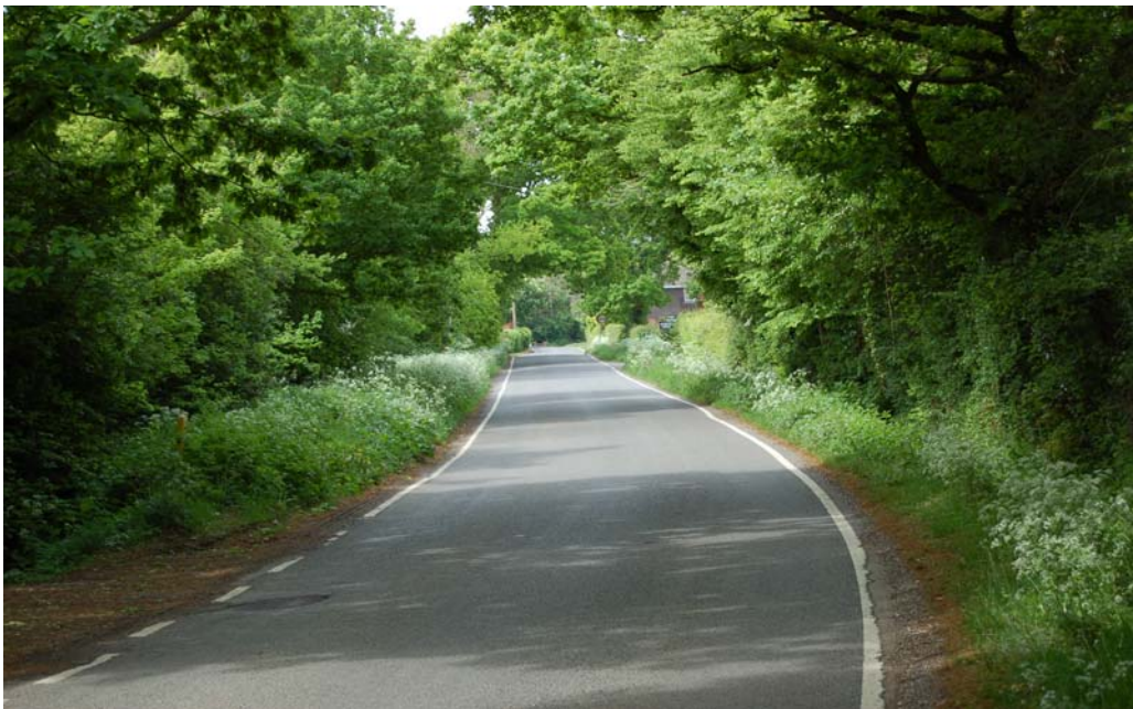
Sector 5 view Chickney Road approach from the east
