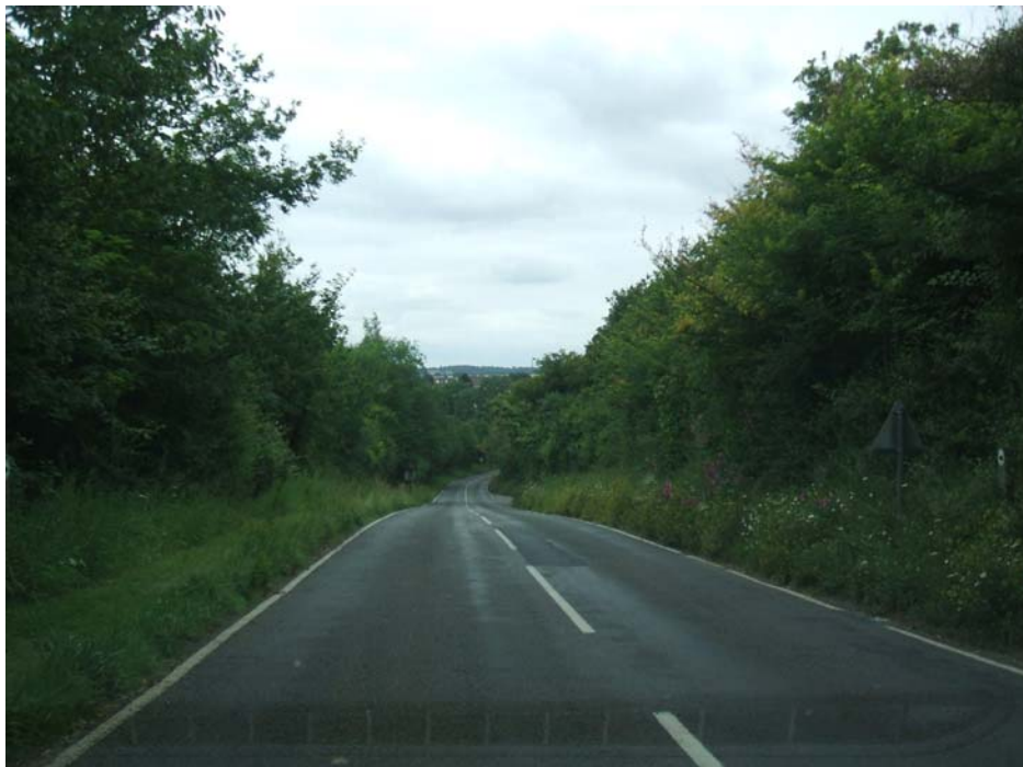
Verges bordering the Debden Road on eastern approach to village
