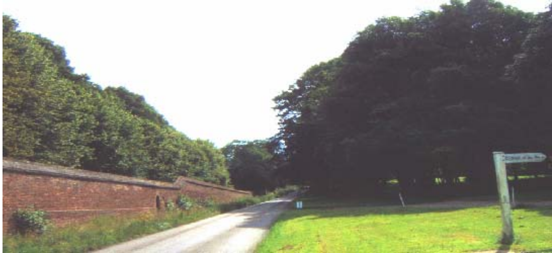
Sector 5 looking east at junction to Audley End village.
