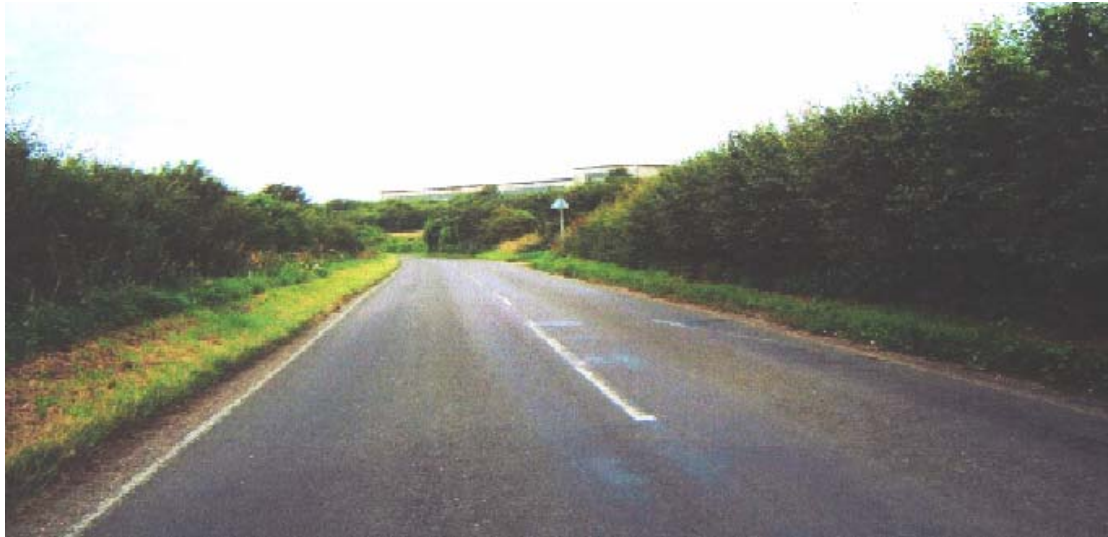
Sector 2 looking west towards Ashdon Road commercial centre.
