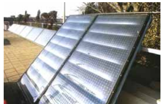
Example of a flat plat solar collector of the kind used for solar water heating or active solar space heating - Flisol
