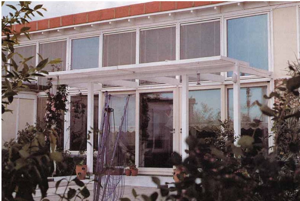
Figure 2-19: Example of a fully glazed Direct Gain Passive Solar Heated House. Solar Courtyard Houses in Milton Keynes Energy World (Fielden Clegg)
