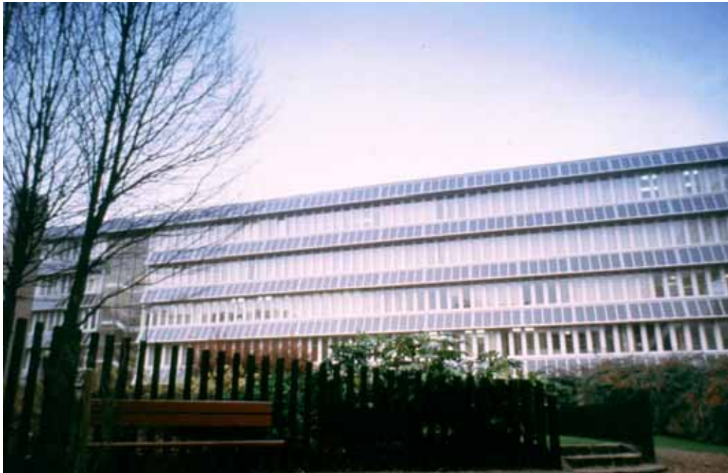
Figure 2-33: PV clad office building at the University of Northumbria. 40 kW peak power.
