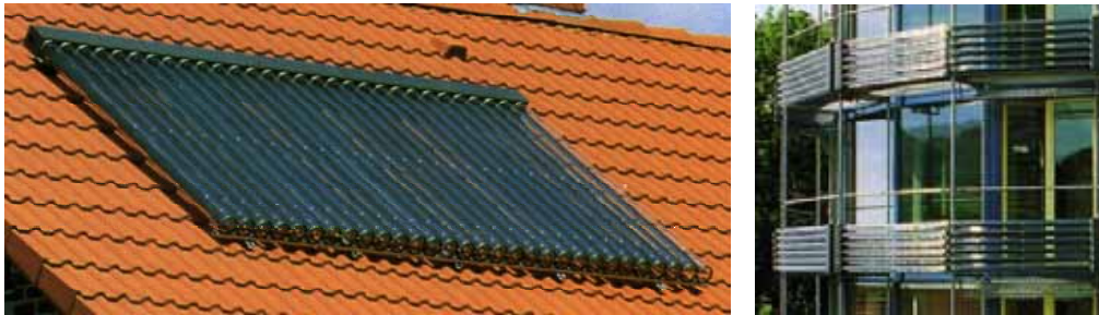
Figure 2-4: Two examples of evacuated tube solar water heating systems.
