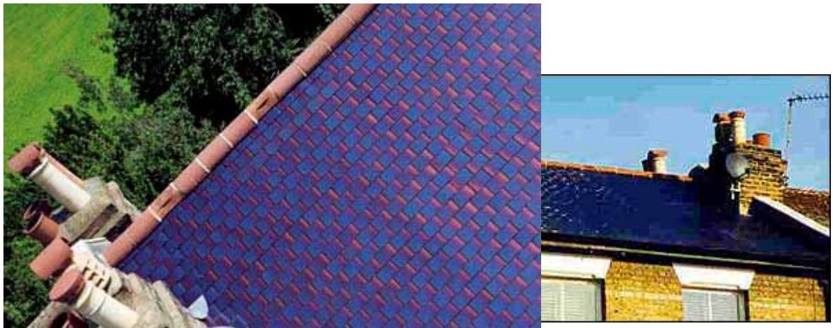
Figure 2-36: Example of a PV roof cladding which mimics roof slates (solar shingles based on ASI-2J) on a house in Richmond (Solar Century)
