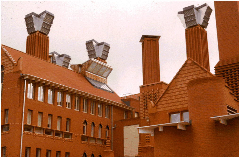
Figure 2-22: Queens Building at De Montfort University which uses cooling towers to passively ventilate and cool the building. Designed by Short Ford & Partners.
