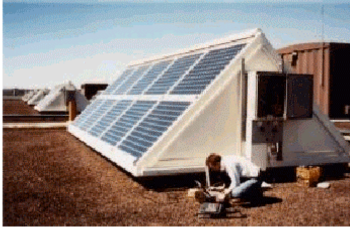
Figure 2-39: PV Clad North-Light Roof-lights. BP Solar.
