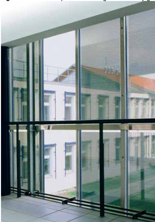
Figure 2-38: 'Tinted' transparent PV/Glazing for PV and daylight provision (Schott)
