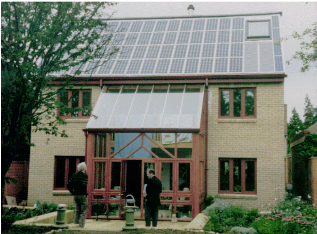
Figure 2-34: PV Modules used a roof covering on the Oxford Solar House. 4 kWp of monocrystalline silicon PV modules. The house also utilises active solar water heating, and passive solar heating via direct gains and from a solar sun-space. (Altechnica)
