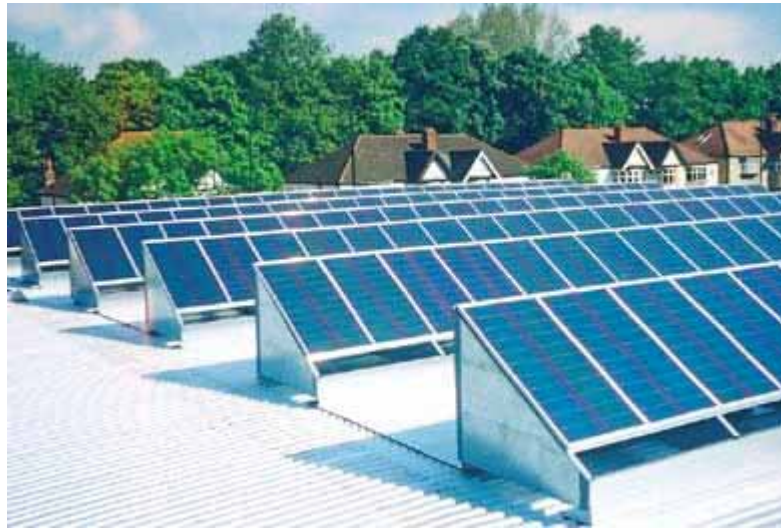
Figure 2-35: An example of PV systems installed on a flat roof. (Solar Century)
