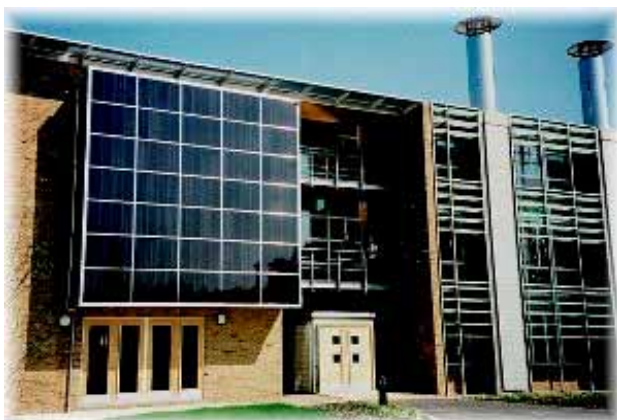
Figure 2-23: BRE Environmental Office which also uses cooling towers. Designed by Fielden Clegg & Partners.
