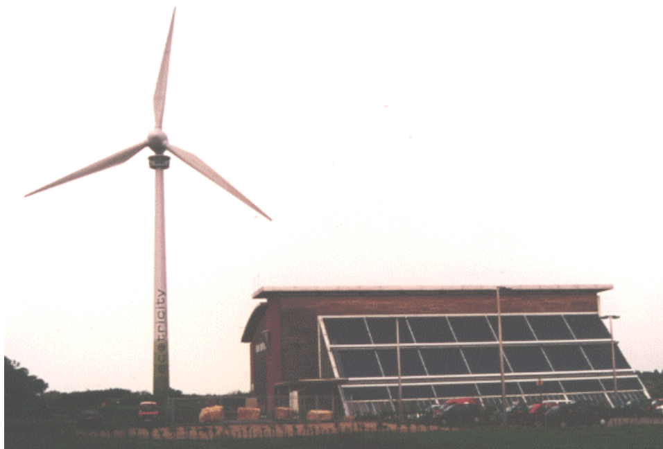
Figure 3-24: 1.5 MW Enercon wind turbine at an environmental centre at Swaffham in Norfolk. (Altechnica)
