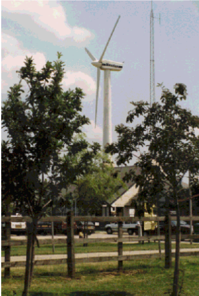
Figure 3-23: 225 kW medium scale Vestas wind turbine at Wood Green Animal Shelter (Altechnica)
