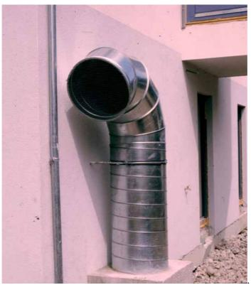
Figure 4-3: Grilled inlet for an Earth Tube/ Pipe. (Altechnica)
