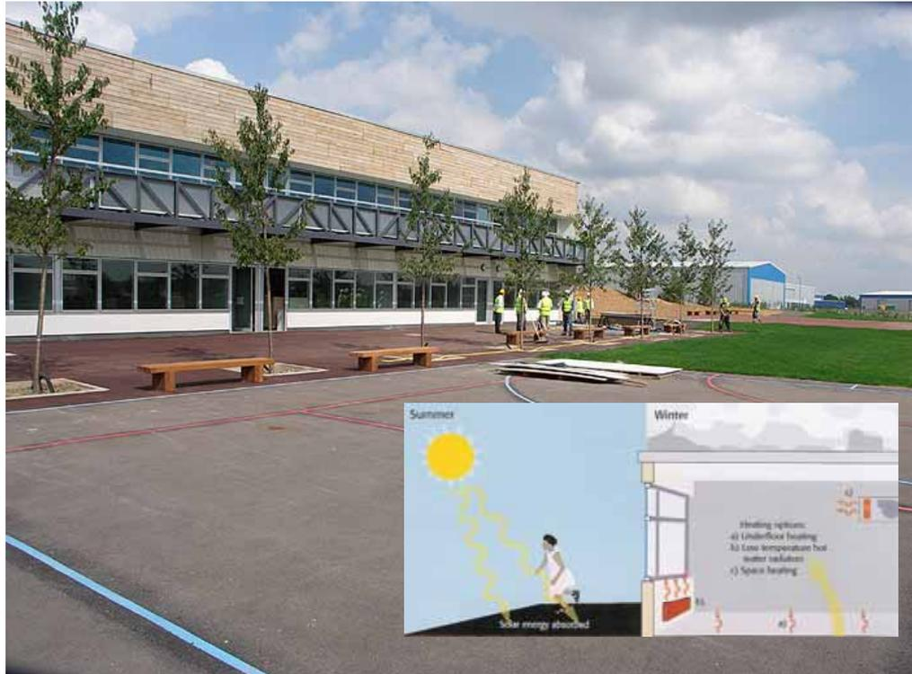
**Figure 4-38:** The ICAX IHT sandwich type system for using a playground for solar-assisted ground coupled energy for heating a school in Hertfordshire. Source ICAX Ltd
