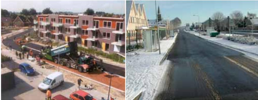
**Figure 4-36:** Examples of the *Road Energy System* + interseasonal energy storage. Heating 70 'care houses' (left) and keeping a Dutch road ice free using the roads as solar collectors (right) . Source Ooms
