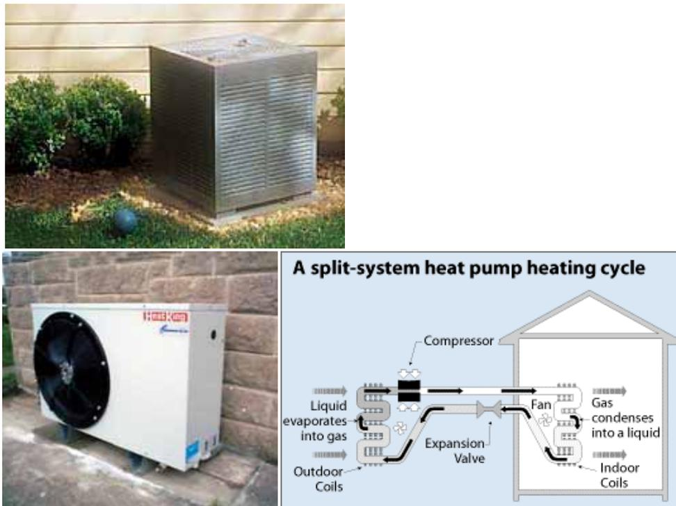
**Figure 4-18:** Two examples of Air Source Heat Pumps (Source Heat King) & Diagram of a Split System Air Source Heat Pump (Source: EERE)
