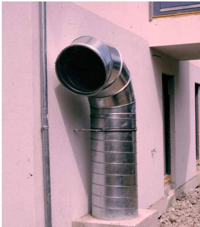
**Figure 4-3:** Grilled inlet for an Earth Tube/ Pipe. (Altecnica)
