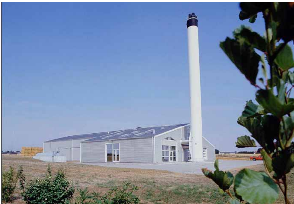
Figure 5-23: Danish Straw fired district heating plant.
