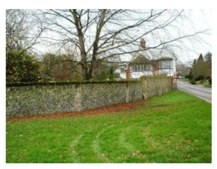
Picture 1.12 Flint boundary wall at the bottom of the Druce
