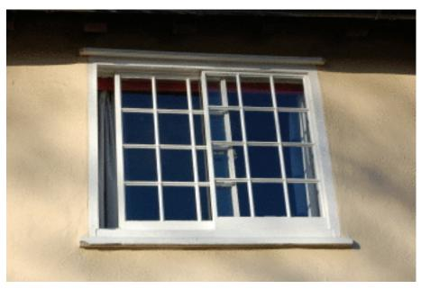
Picture 1.8 Sliding horizontal sash window on the Guildhall, Church End
