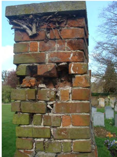
Picture 1.18 Northern boundary wall to church, urgent repairs needed
