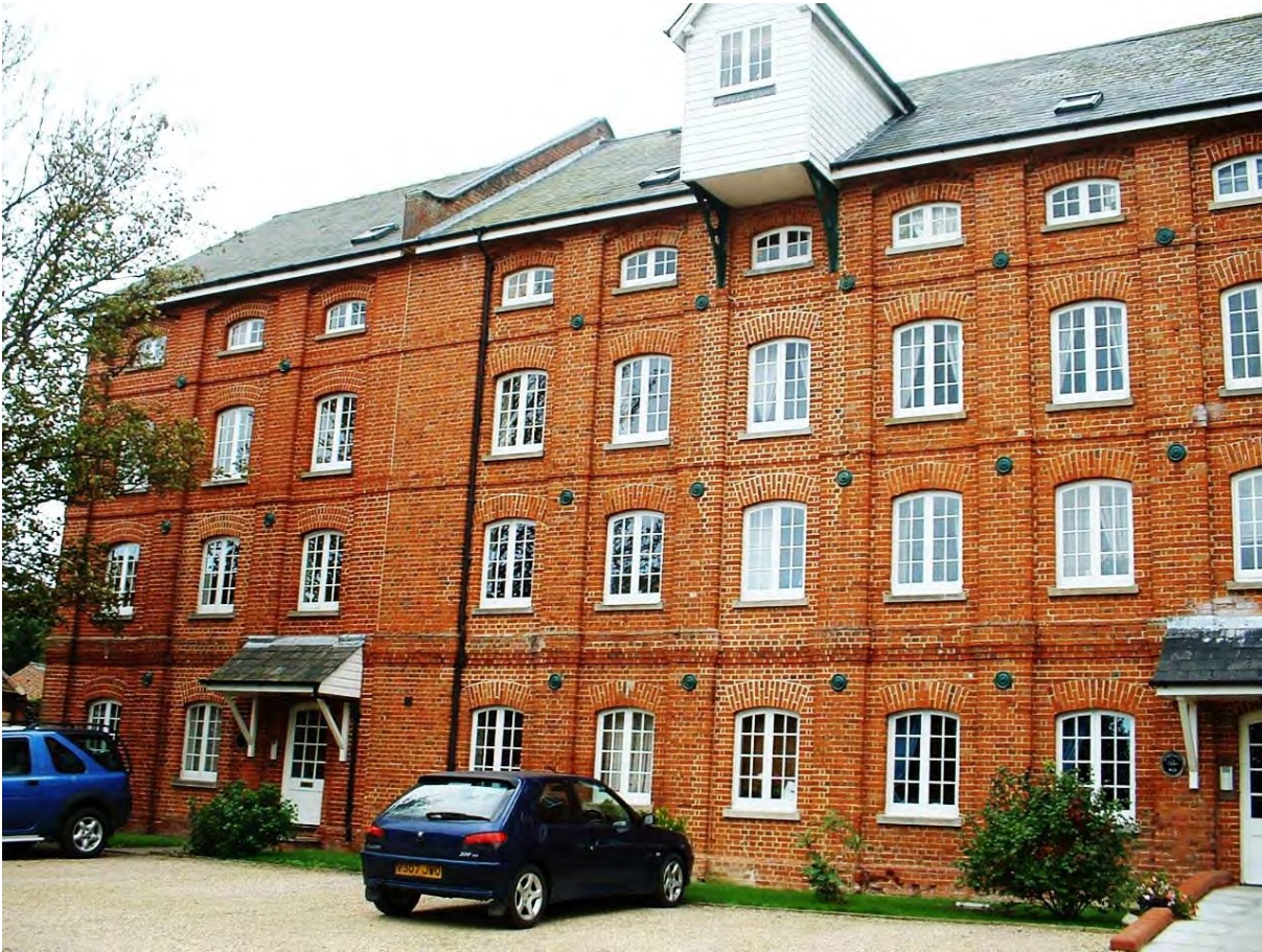
Picture 1.19 Kings Mill converted to flats
