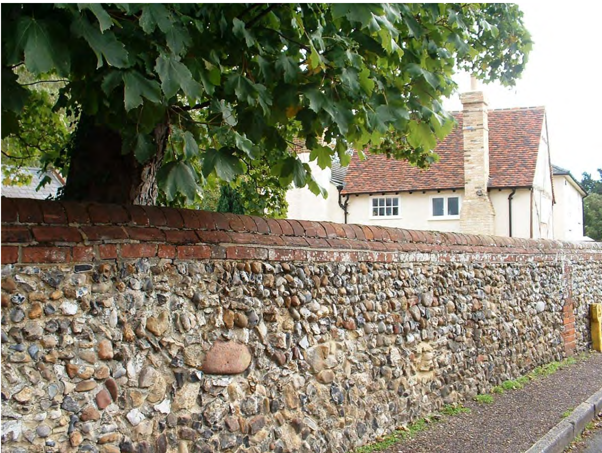
Figure 1.2 Curtilage wall to listed building, The Dalles
