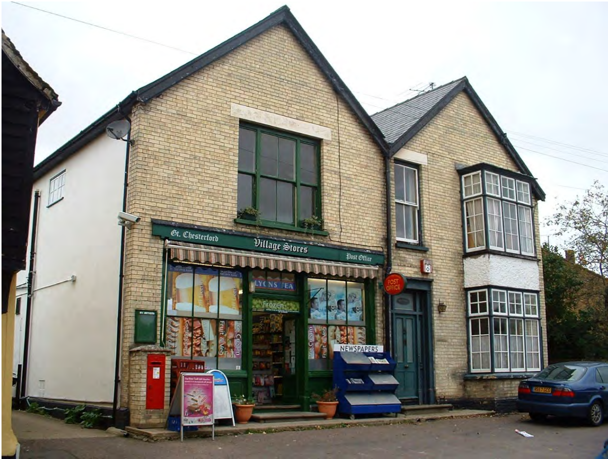
Picture 1.11 Little chnged present view of Post Office building
