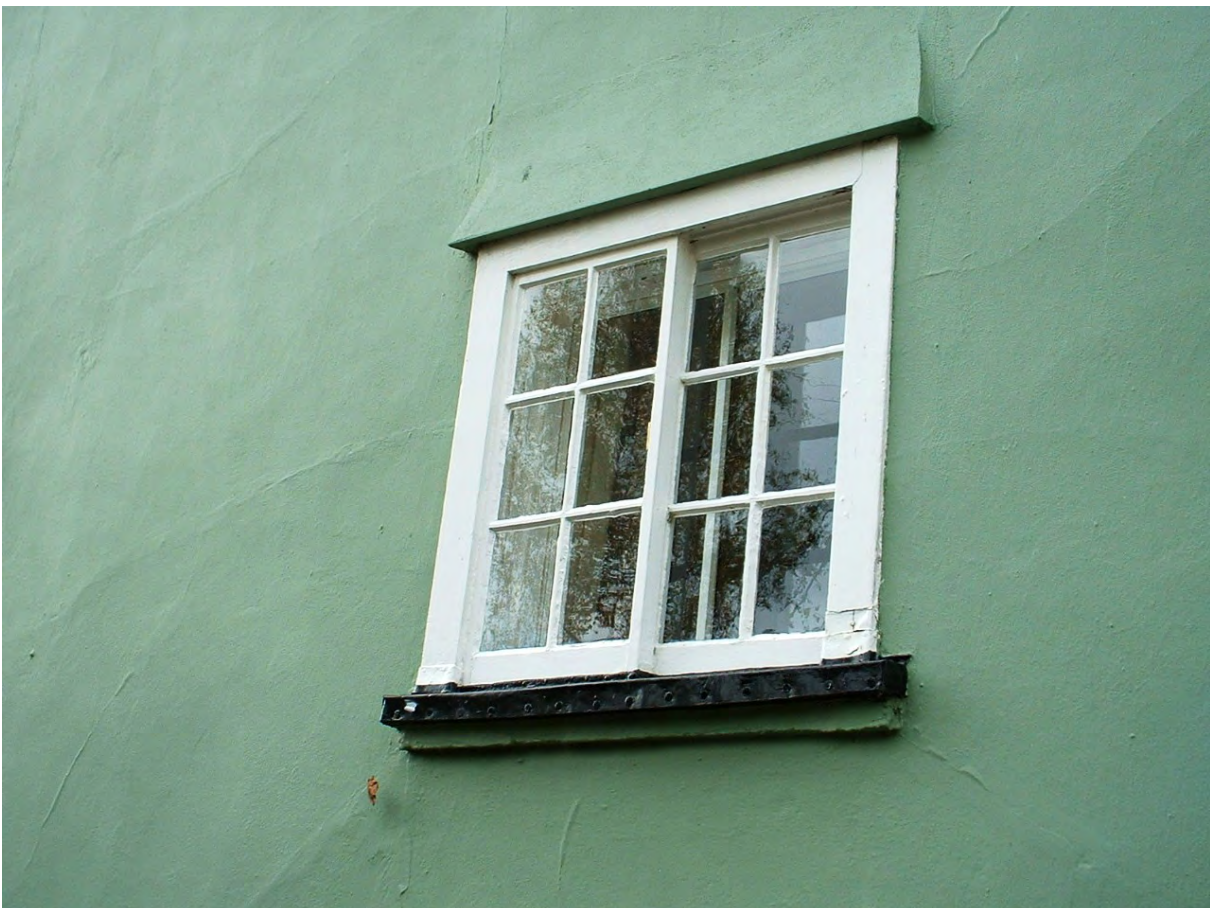
Figure 2.2 Quality horizontal sliding sash window
