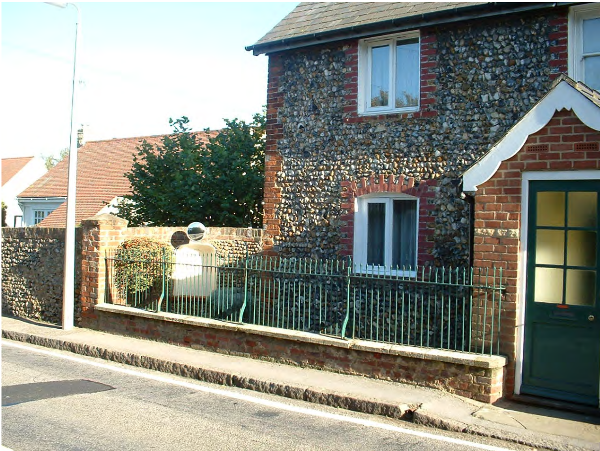
Figure 2.3 Distinctive railings to be protected
