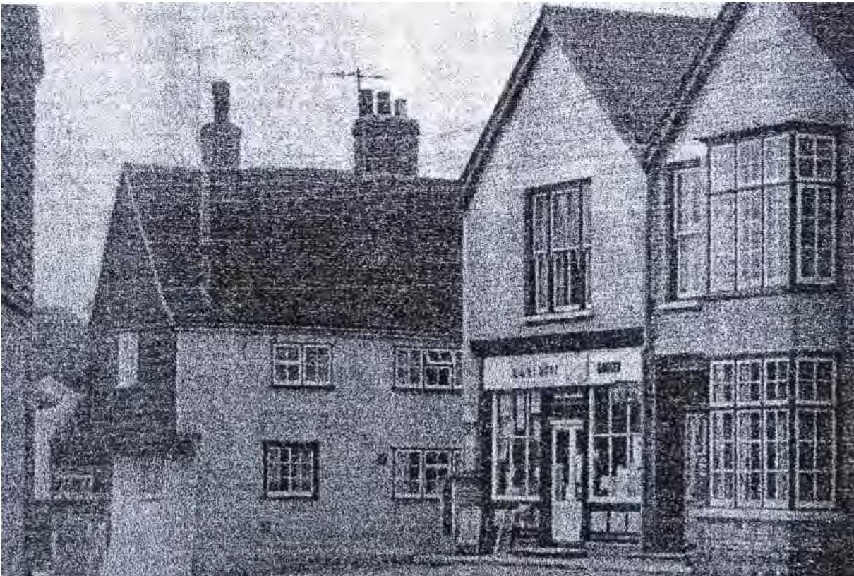
Picture 1.10 Historic view of Post Office building
