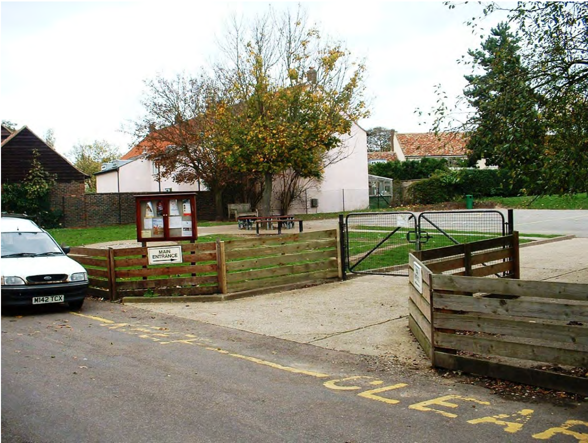
Picture 1.16 Detracting fencing at Primary School
