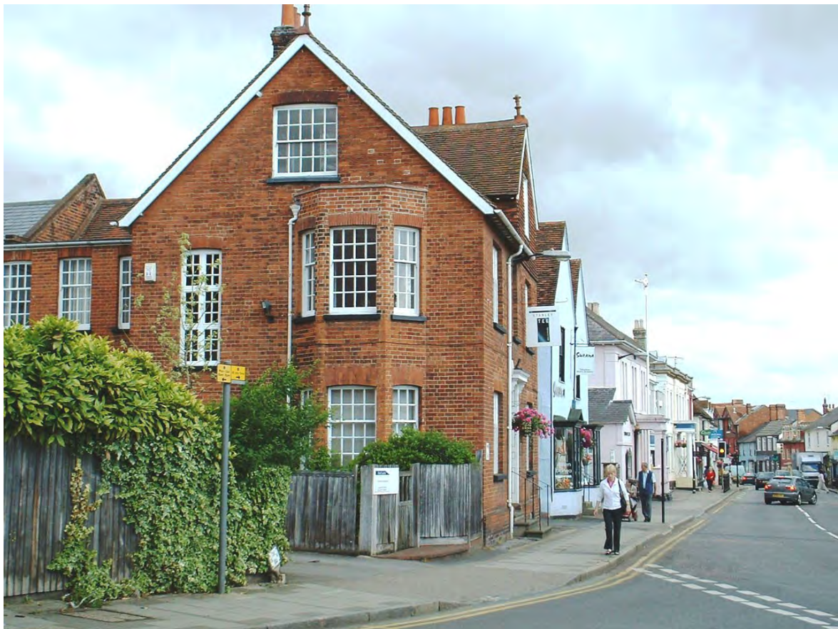
Picture 1.8 No 42 High Street, an unlisted building of quality
