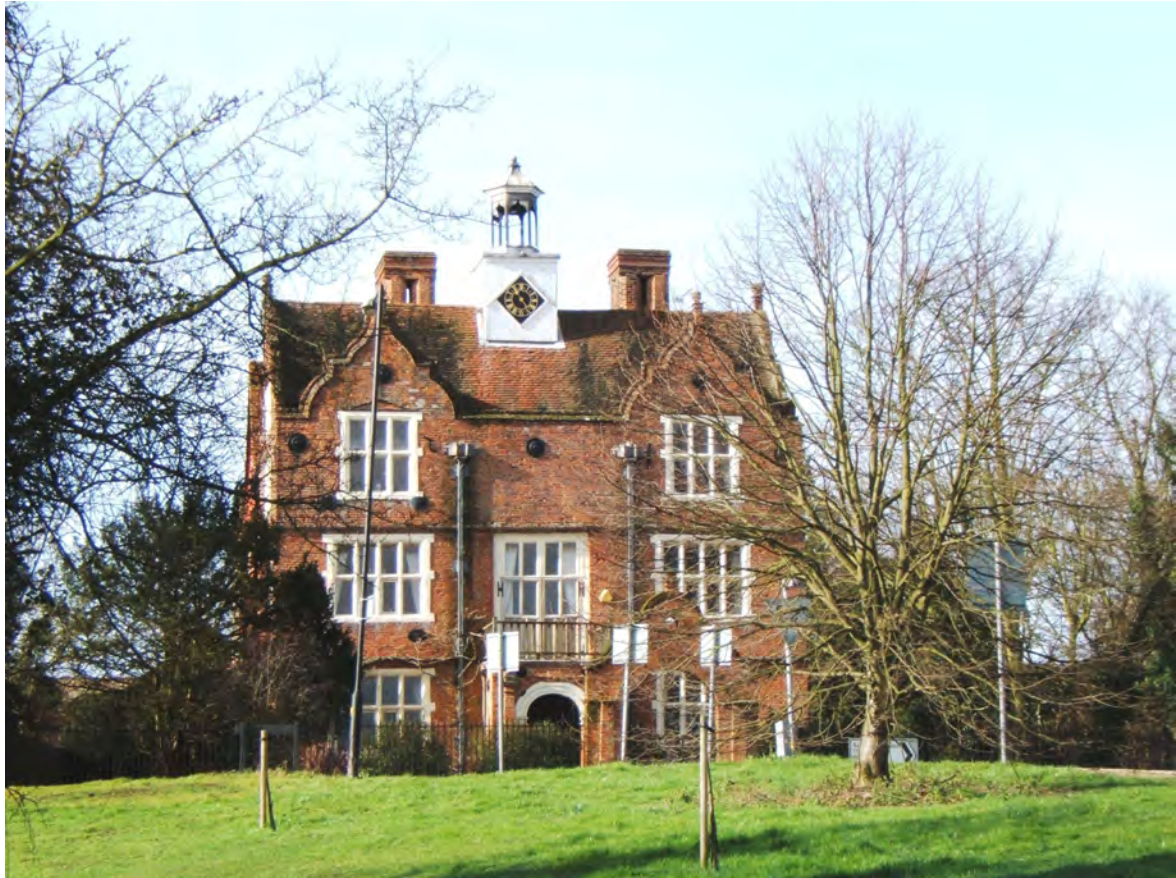
Picture 1.15 Clock House, Beaumont Hill, listed Grade I
