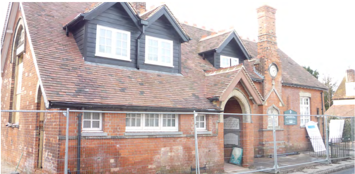
Picture 1.12 Former Memorial School, with works ongoing
