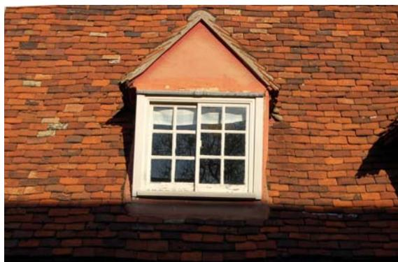
Picture 1.6 Dormer window with horizontal sliding sash,
