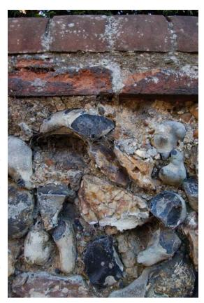
Picture 1.5 Flint wall with half round brick cap at Forge Cottage
