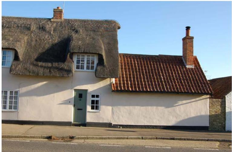
Picture 1.1 Thatch and pantiles on Wheelwright’s Cottage
