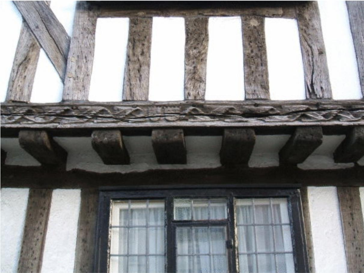
Picture 1.7 The Old Vicarage, detailed carving on timber frame
