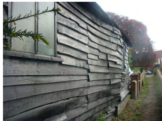
Picture 1.14 Weatherboarded barn of historic value within curtilage of the Old Vicarage
