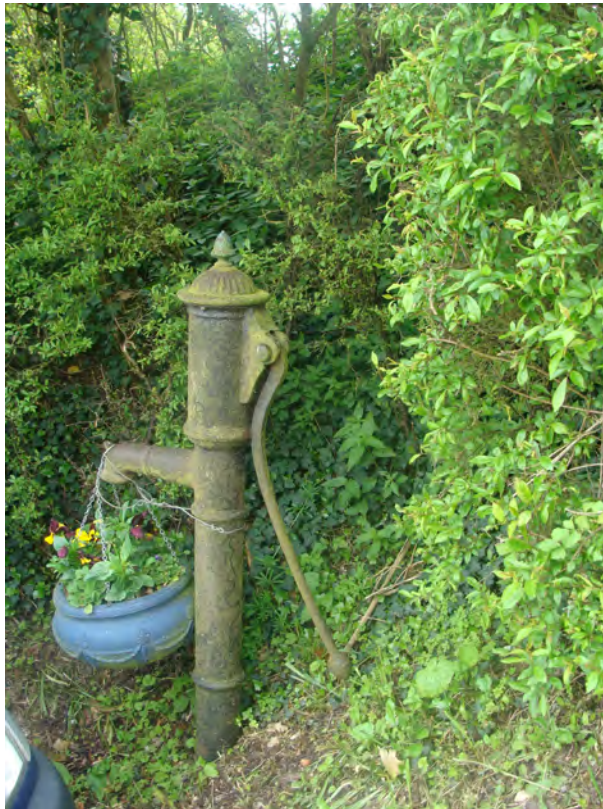
The 19th century cast iron pump at Prince's Well needs repainting. It is a possible candidate for formal listing (left) and (right) another 19th century pump in need of sensitive repair
