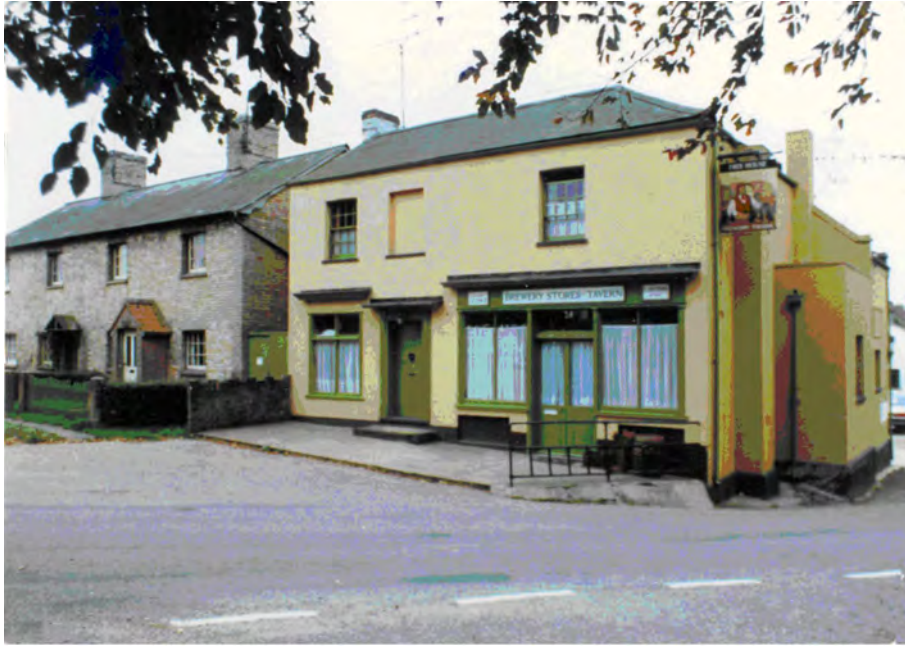
Picture 1.2 Traditional village shop and residence, mid/late 20th century, additional use as Brewery Tavern and enlarged window to left added. Also note porches of differing styles and scales added to adjoining 19th century terrace
