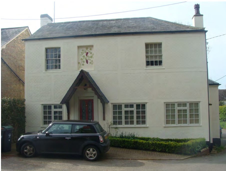
Picture 1.3 The building today, original commercial window detailing replaced and large central porch added. Change of use may have been inevitable but a more appropriate design solution retaining some original features would have been possible
