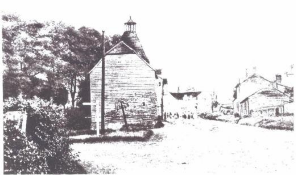
Picture 1.16 Historic View of Church End towards Red Lion with Malttings in foreground
