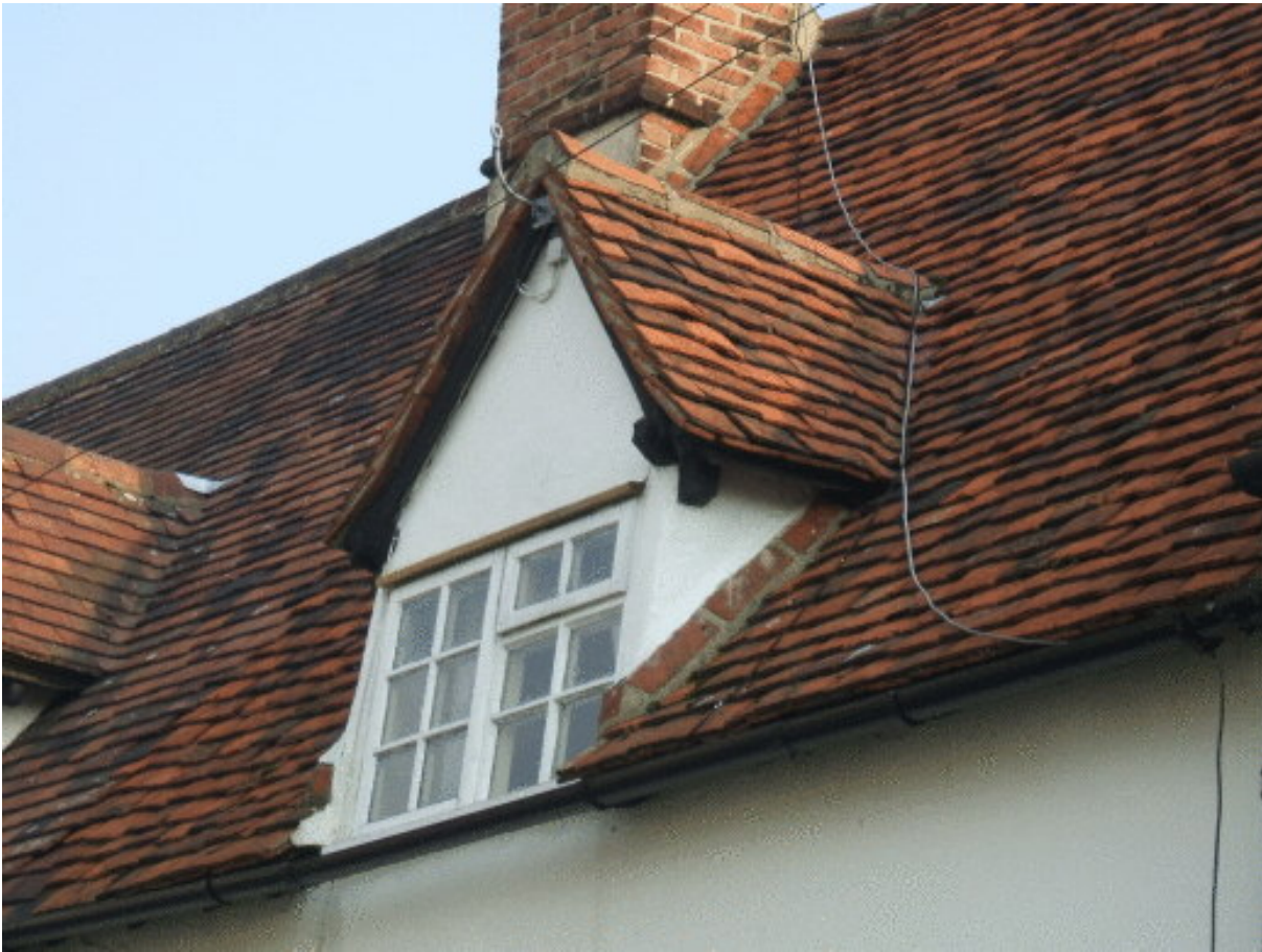
Picture 1.7 Typical small dormer
