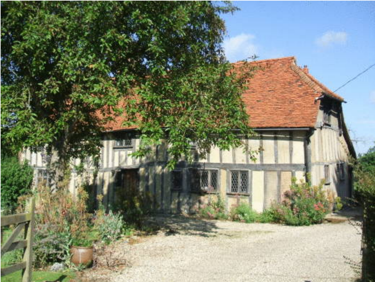
Picture 1.26 Tan Farmhouse, a superb Medieval building
