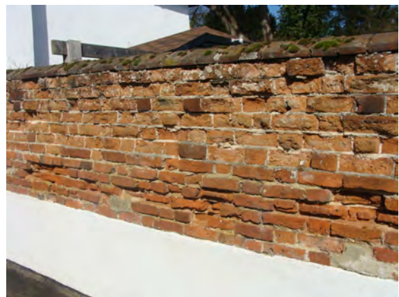
Picture 1.23 Red brick wall in need of restoration to Candle Cottage in strategic location on Stoney Lane
