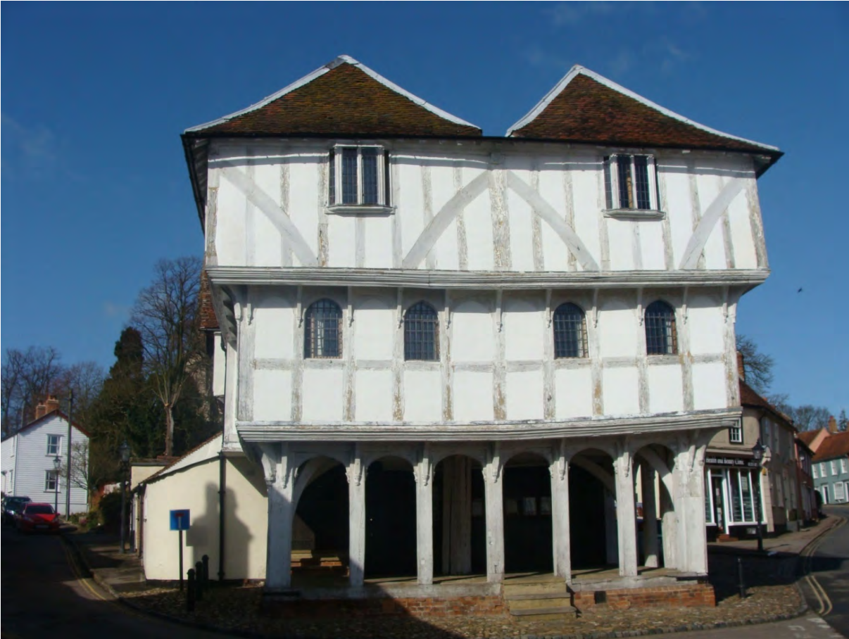
Picture 1.15 The Grade I Guildhall
