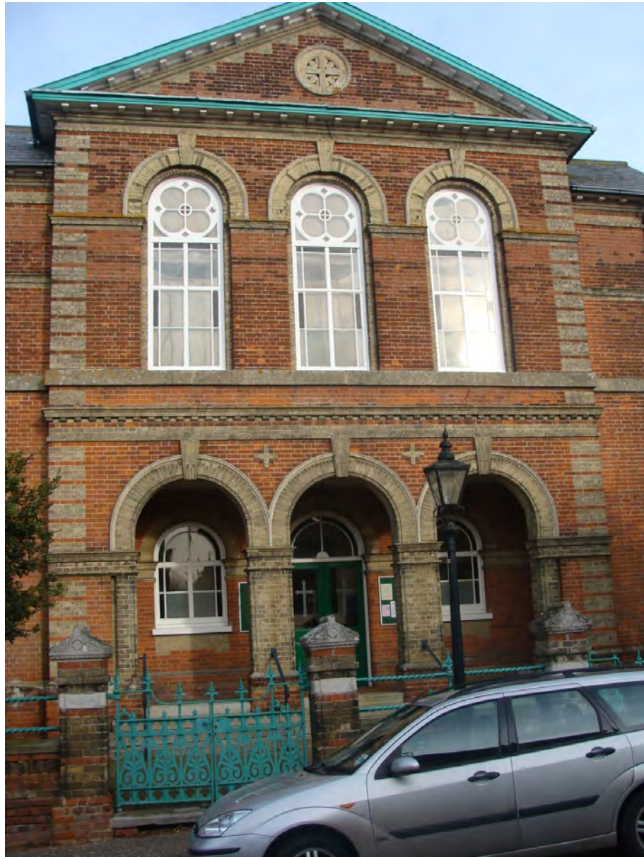
Picture 1.19 United Reformed Church, essentially 19th century in character, a key building in the streetscene
