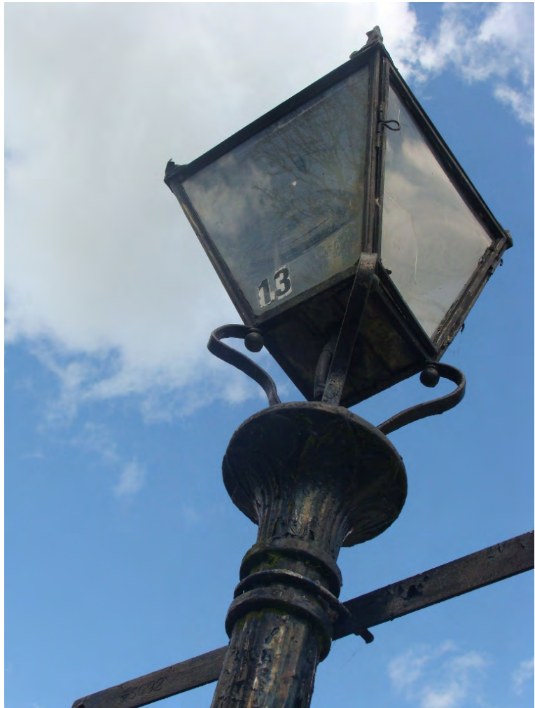
Picture 1.2 Thaxted is lucky in having a considerable number of historic street lamps; many columns are in need of repainting
