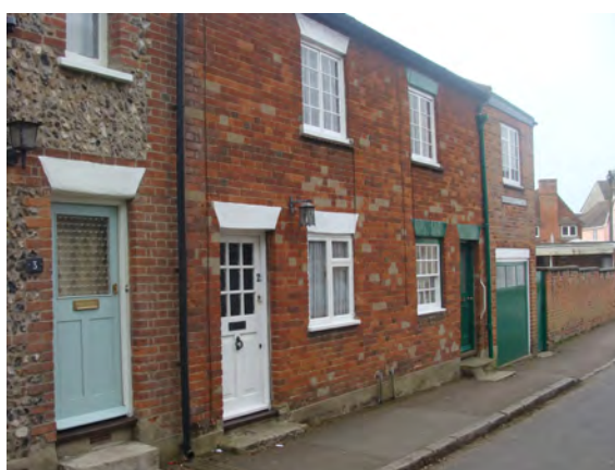
Picture 1.5 Bridgefoot Cottages; a variety of windows, doors and extensions adversely affect their historic character
