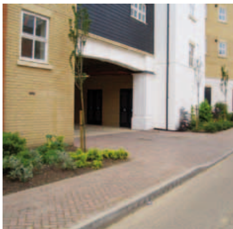
Undercroft secure parking (gated entry).
