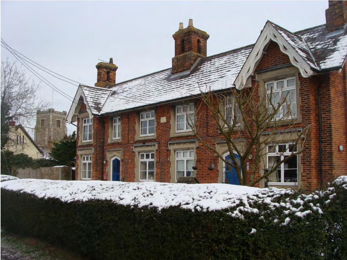
Picture 1.12 Former late 19th century almshouses with several distinctive architectural features worthy of preservation, possibly by Article 4 Direction subject to further consideration and notification
