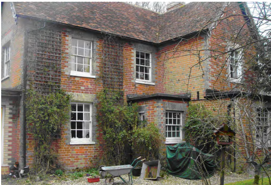
Picture 1.14 Trevor House Windows and other selected architectural detailing which may be protected by an Article 4 Direction subject to further consideration and notification
