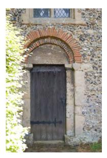
Picture 1.12 Roman brick re-used in the arch of the door on the west tower to St Mary's Church
