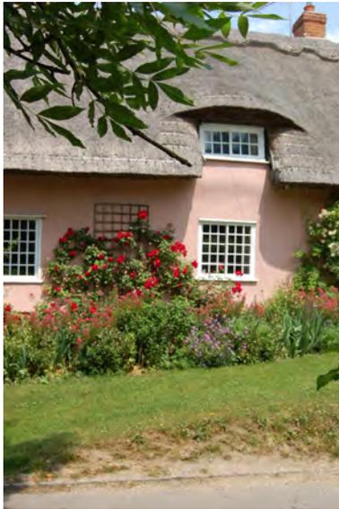
Picture 1.11 Thatch, horizontal sliding sahes and delicate colour-washed plaster in Church Path
