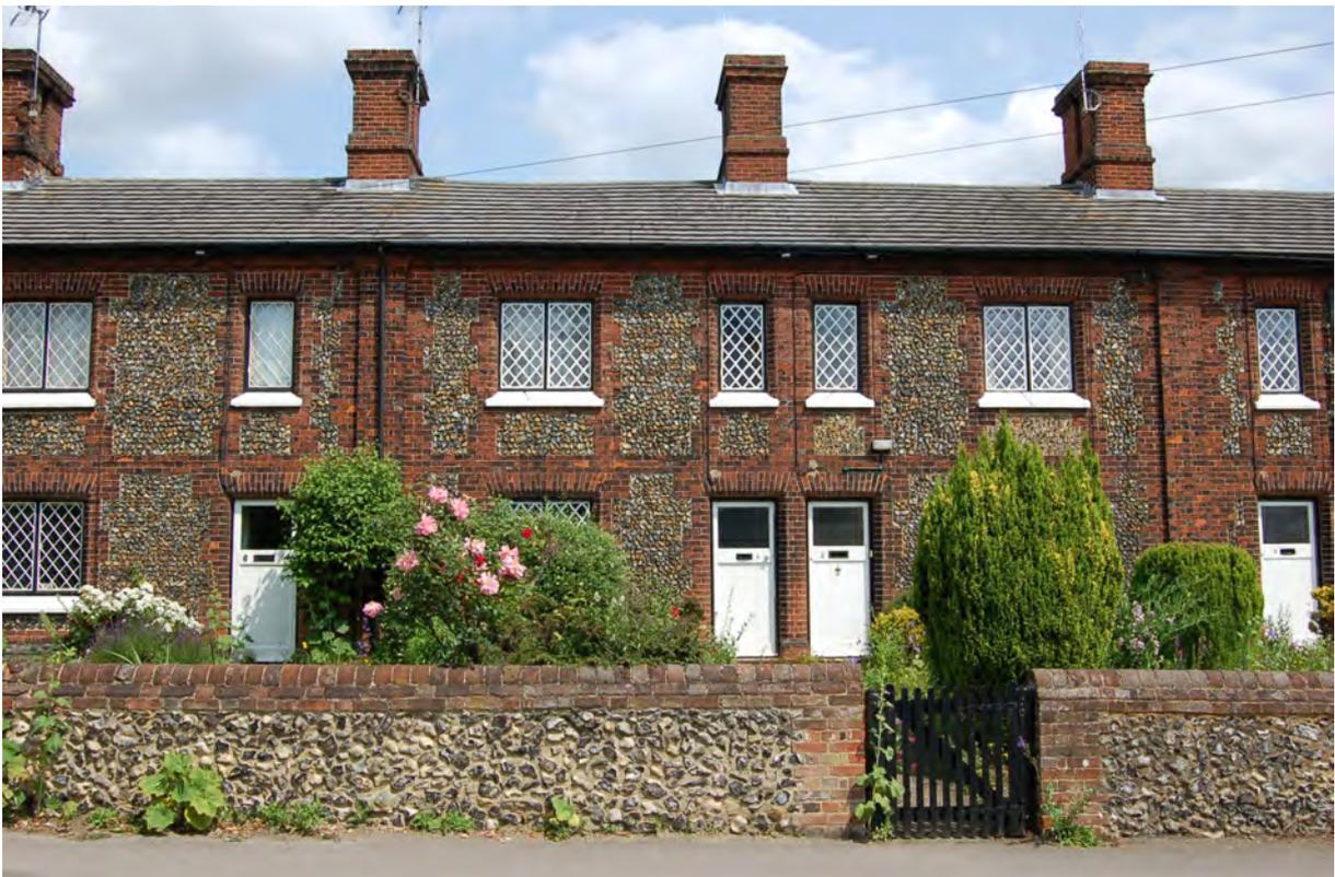
Picture 1.21 Railway Cottages. The combination of flint panels, high quality brick detailing and lattice windows makes a very pleasing and important run of buildings at this entrance to the Conservation Area
