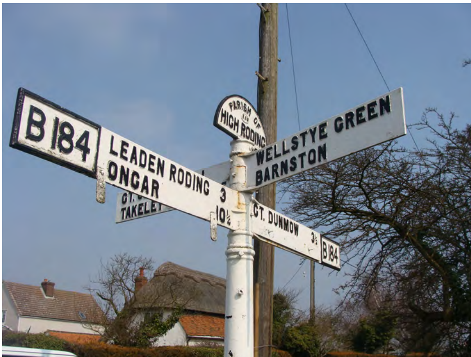
Picture 1.20 Good quality four way metal directional sign, supporting post of which needs repainting. An important feature most worthy of retention
