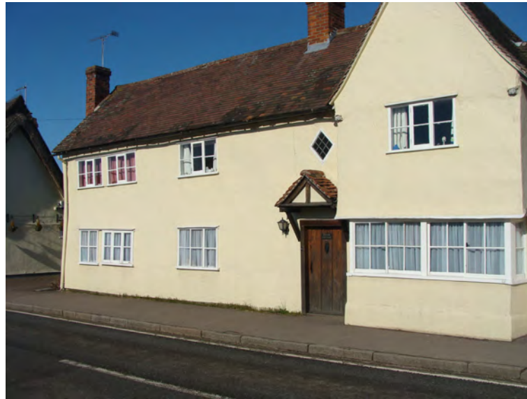
Picture 1.5 Salem Cottage, originally a Hall House dating from about 1400. The roof was originally thatched but replaced with tiles following a fire in 1973
