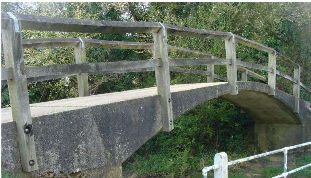
Picture 1.21 Delicately proportioned bridge crossing River Chelmer. It and metal safety railings would benefit from maintenance and repainting.
