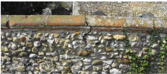
Picture 1.14 Wall surrounding graveyard, small area in need of repair.
