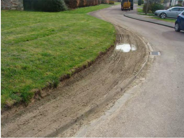
Picture 1.18 Badly eroded edge to open space fronting south elevation of church. A sensitive resolution of this problem would be beneficial
