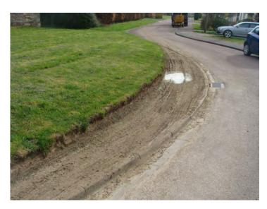
Picture 1.18 Badly eroded edge to open space fronting south elevation of church. A sensitive resolution of this problem would be beneficial
