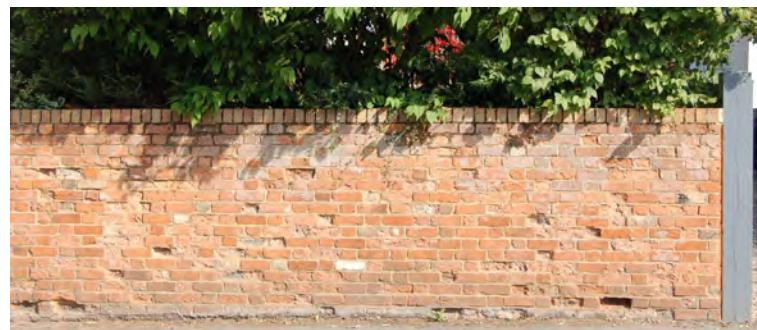
Picture 1.20 Spalled brickwork on the wall between Chestnut House and No.2 The Cottages detracts from the overall quality of the streetscene.
