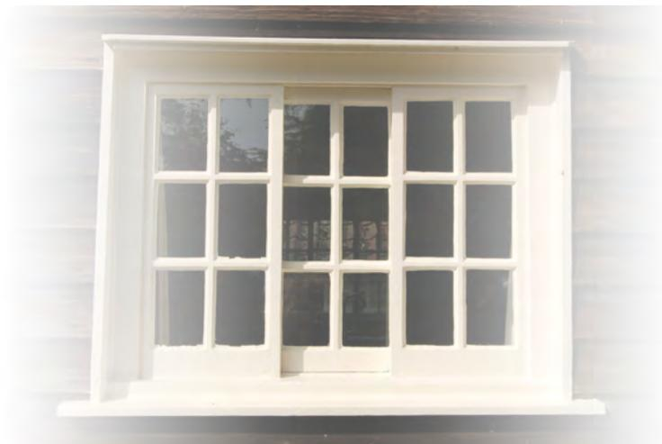
Picture 1.15 Horizontal sliding sash at Beam Ends
