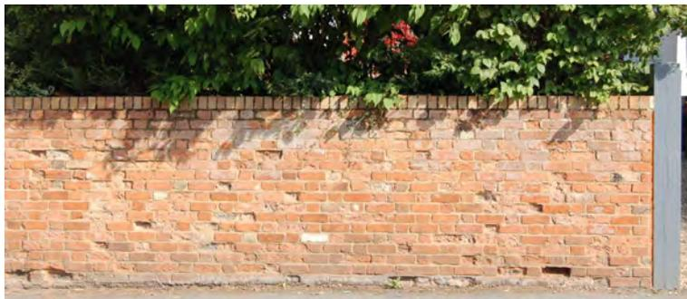
Picture 1.20 Spalled brickwork on the wall between Chestnut House and No.2 The Cottages detracts from the overall quality of the streetscene. Remedial action would be desirable
