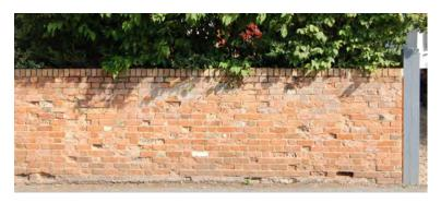
Picture 1.20 Spalled brickwork on the wall between Chestnut House and No.2 The Cottages detracts from the overall quality of the streetscene.
