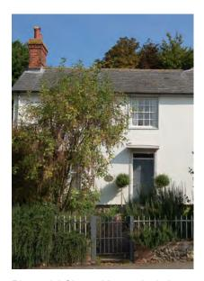
Picture 1.6 Slate, white-washed plaster and simple iron railings on a half height flint wall in Linton Road
