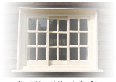
Picture 1.15 Horizontal sliding sash at Beam Ends
