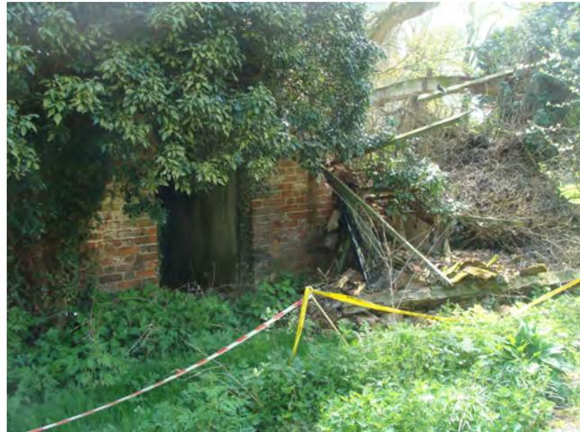
Picture 1.15 Same derelict building, northern elevation. As can be seen southern end is probably incapable of meaningful restoration
