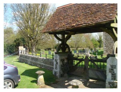
Picture 1.13 19th century church boundary wall and Lychgate, the wall is in need of repair in places
