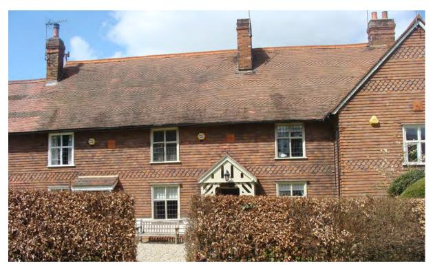
Picture 1.12 Nos. 1,2 and 3 Church End, 17th century in origin with distinctive 19th century scalloped tile detailing to walls and roof
