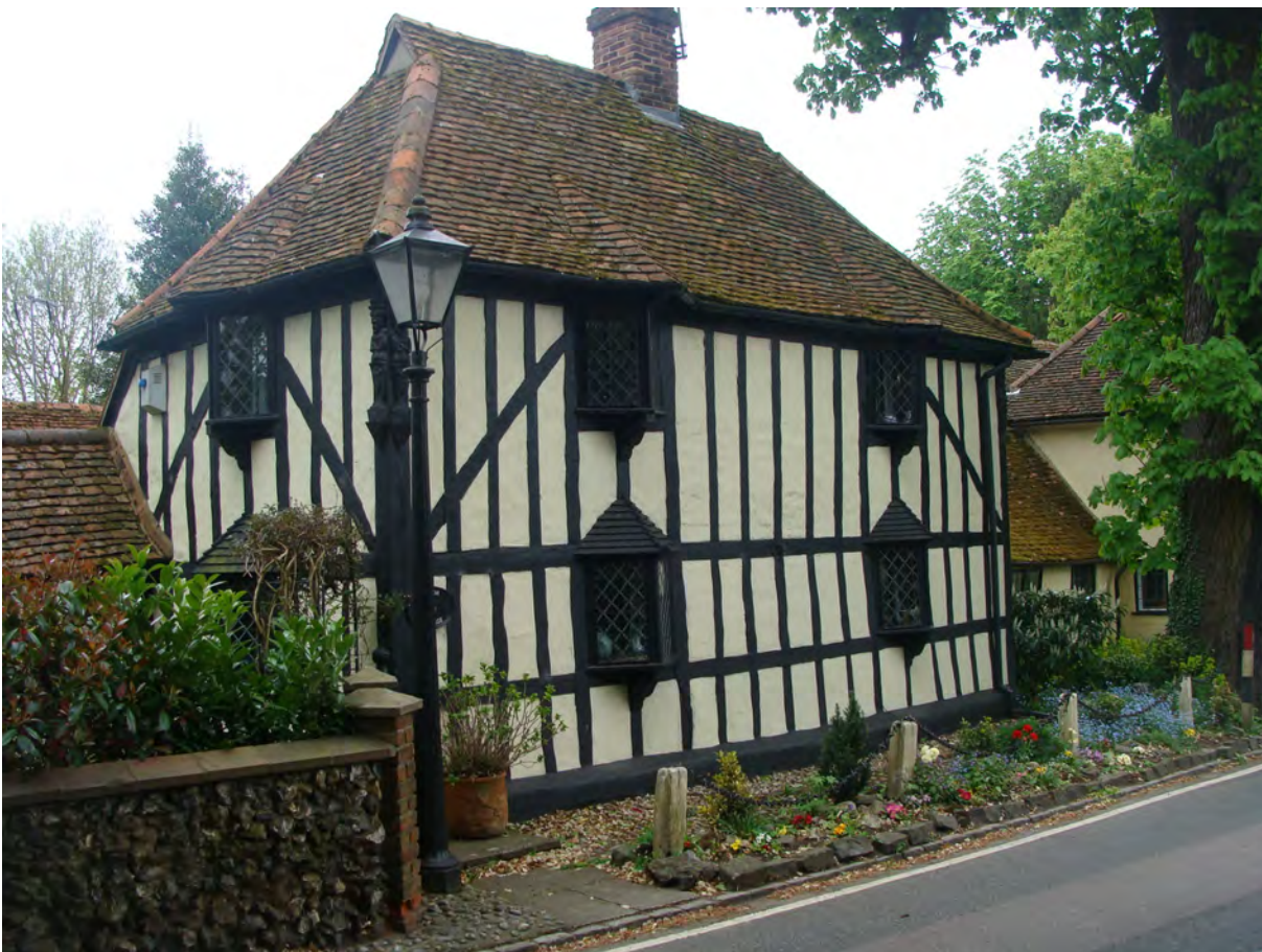
Picture 1.8 Tudor Cottage, a Listed Building dating from the 15th century, prominent in the street scene
