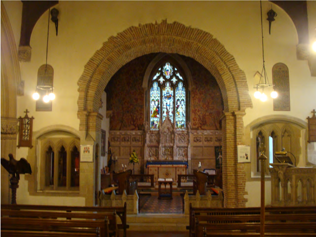
Picture 1.10 The early Norman chancel arch in St Giles church built entirely of Roman bricks
