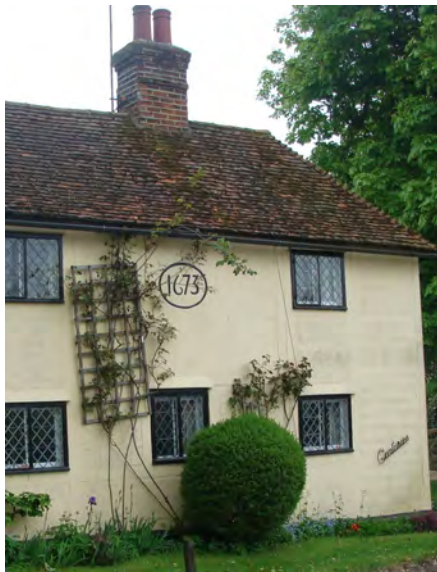
Picture 1.3 Pargetting, colour-washed plaster and simple detailing on Centuries In Church Road
