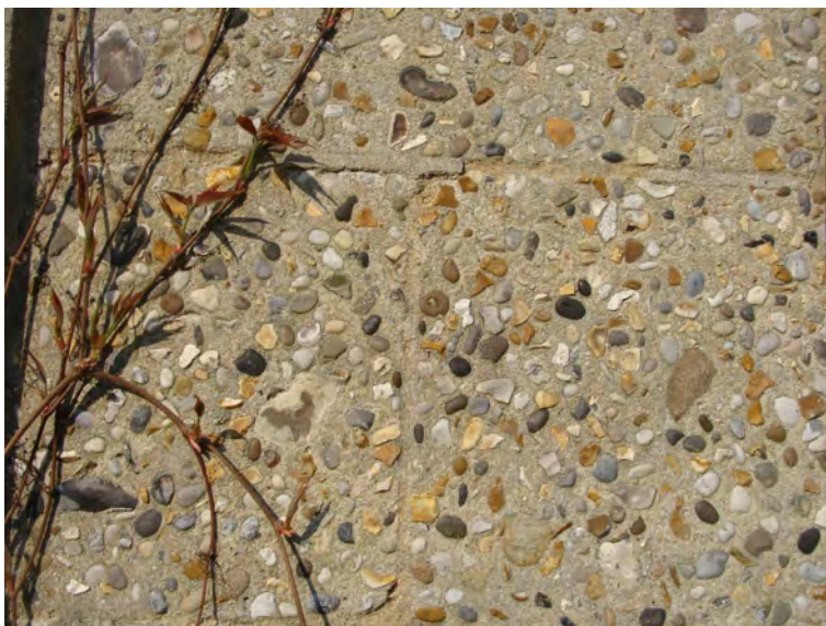
Picture 1.18 Glebe House, Church Road. An unusual late 19th century building constructed of or faced with concrete and exposed aggregate block detailing. Unusual and most worthy of retention
