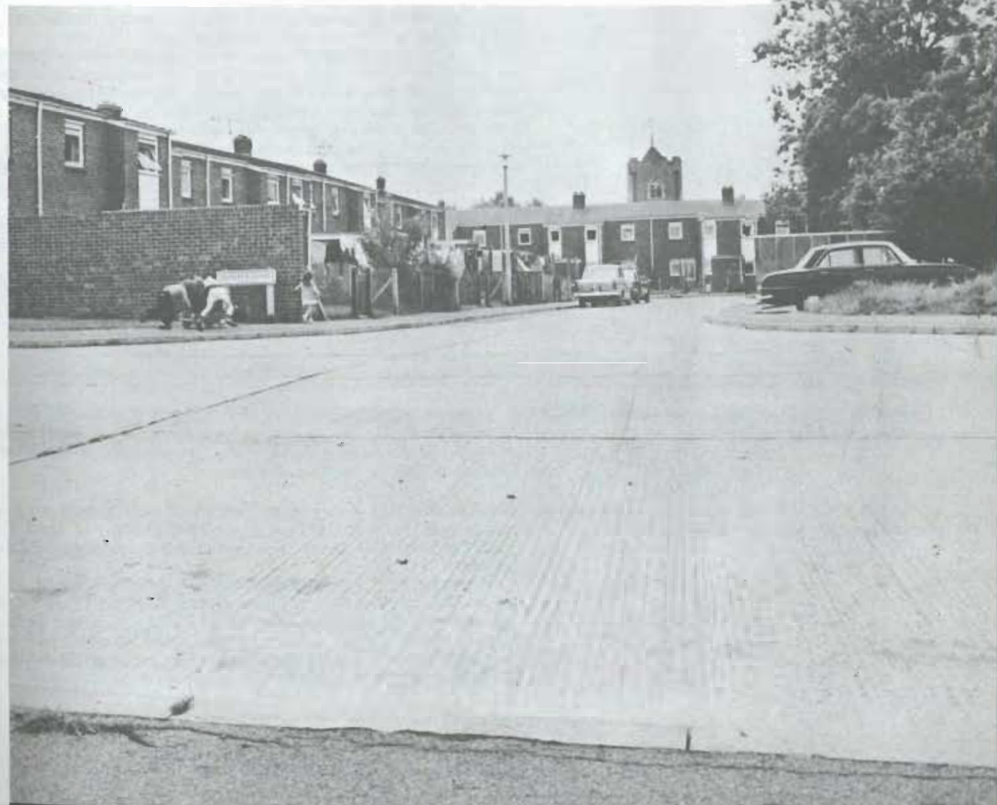
1.0 e Rear access housing, Boreham Village, Essex.
