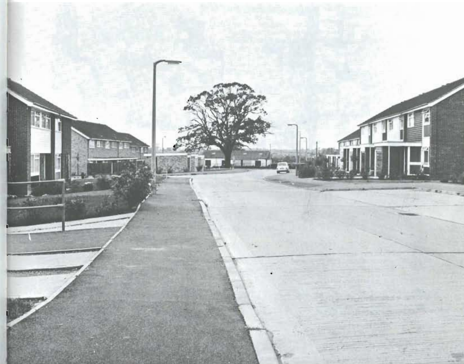
PHOTOGRAPH - Typical Suburban Scheme
