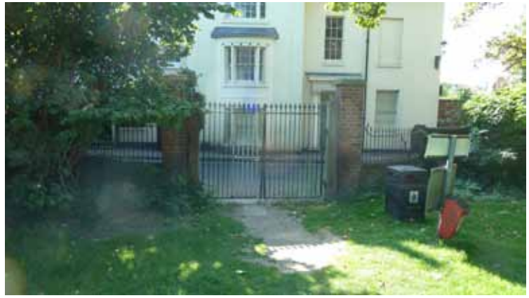
Interior view of gate, existing
