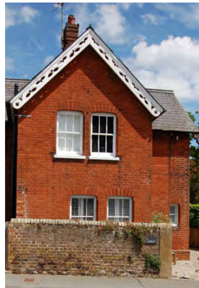
Picture 1.5 Decorative barge boards employed to dramatic effect under a slate roof on West Lodge - a building formerly associated with the Hargrave Park estate.
