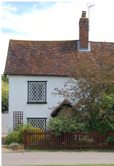
Picture 1.4 Clay tiles, white-washed plaster and distinctive diamond pane windows behind a simple picket fence on Laundry Cottage.
