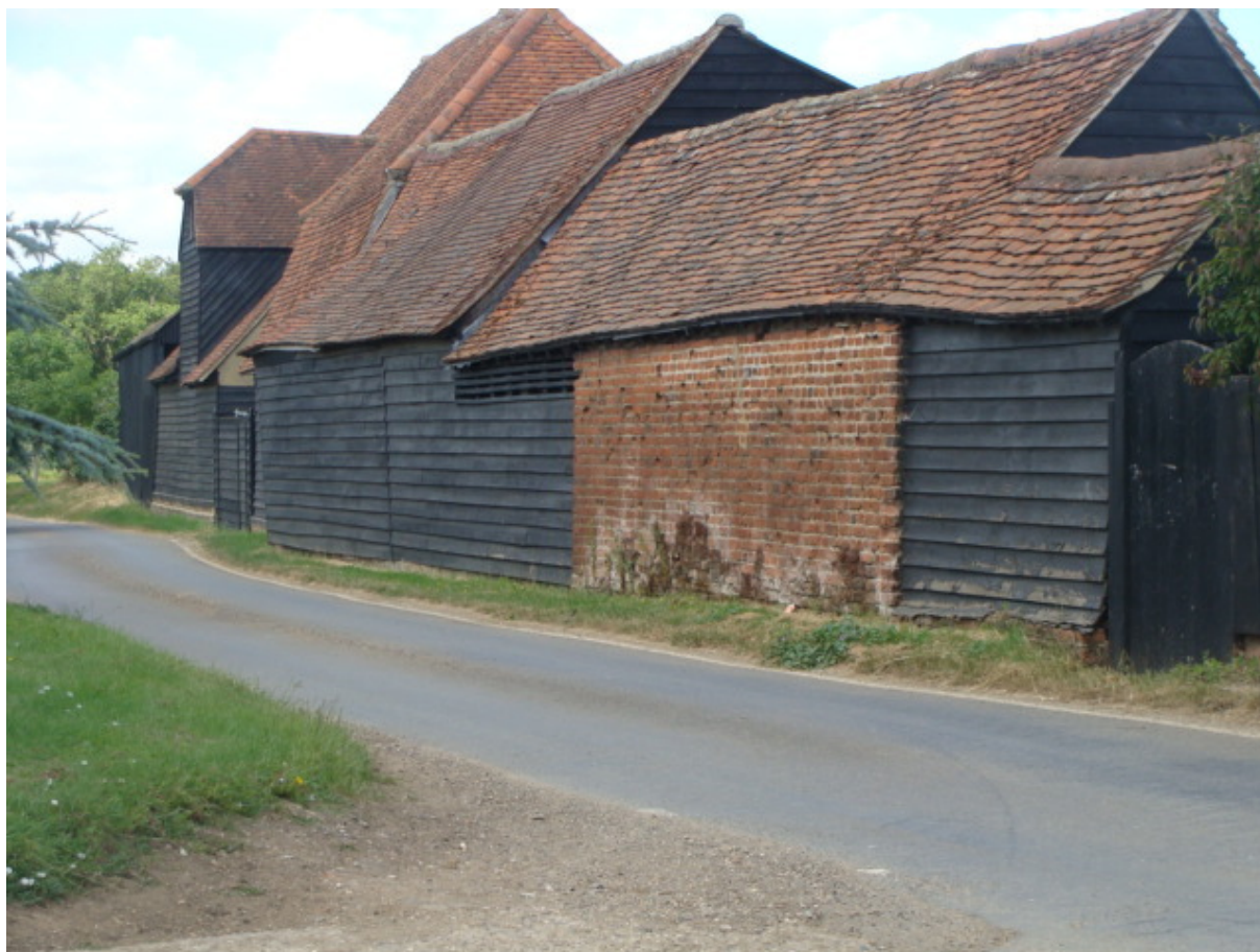
Picture 1.4 Range of timber-framed outbuildings to west of Home Farmhouse whose varied roofscape adds character and diversity to this part of the street scene.
