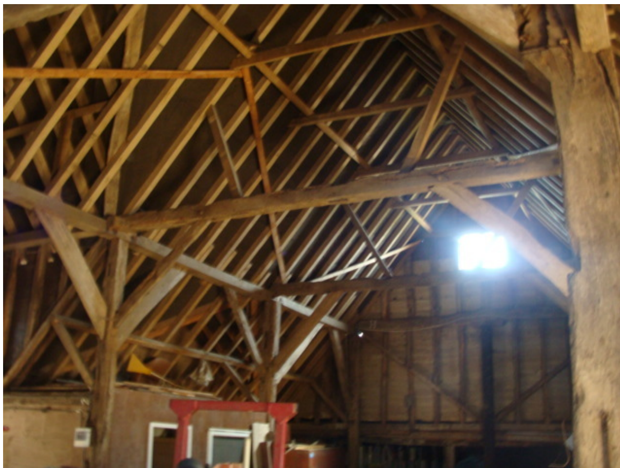
Picture 1.6 Interior of reconstructed barn being that to the south east of Upper Farmhouse. Original structure burnt down in 1980.
