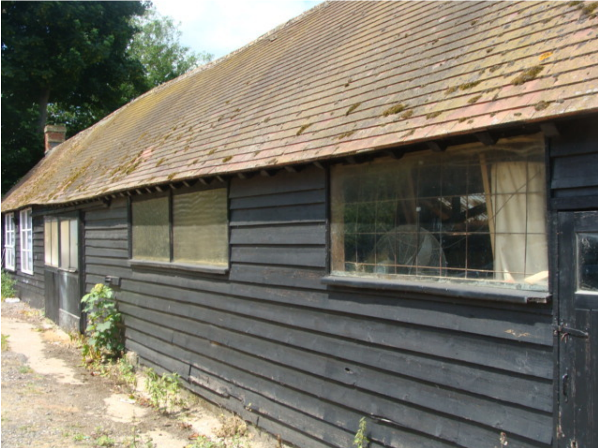
Picture 1.9 Curtilage listed storage building to south west of The Castle, worthy of retention.
