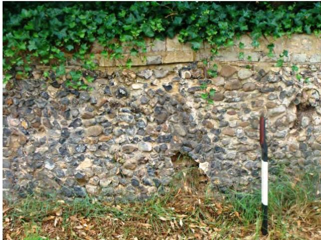
Picture 1.25 Selected areas of important wall to boundary of the Old Vicarage are in need of repair.
