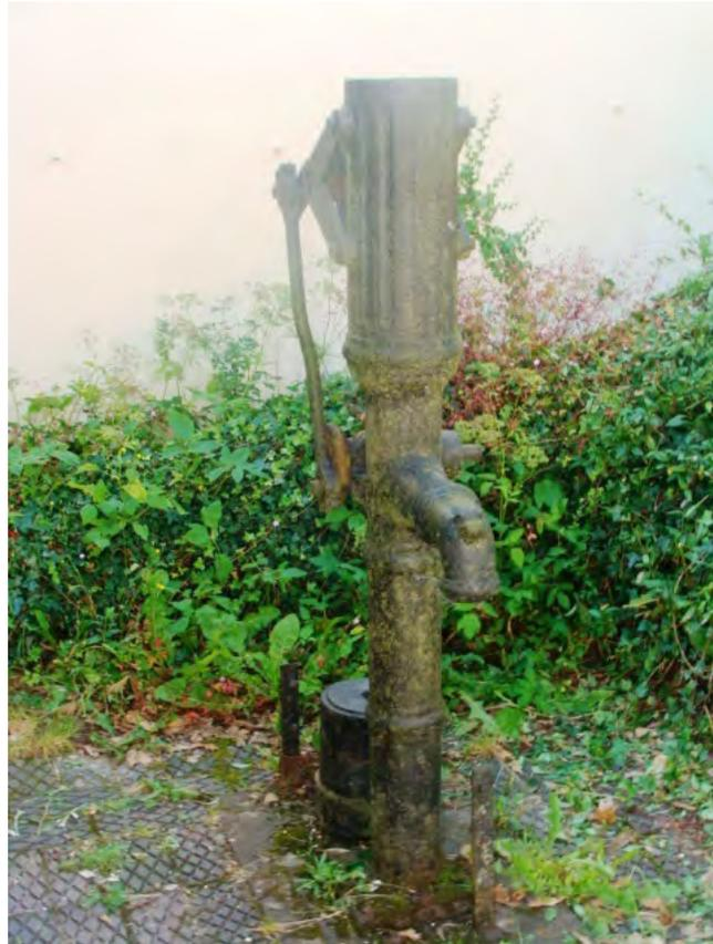
Picture 1.30 Traditional village pump that is very much part of the local history and in need of some restoration. Various levels of restoration possible but an immediate improvement could be achieved by removing weed growth and re setting slate paviours.
