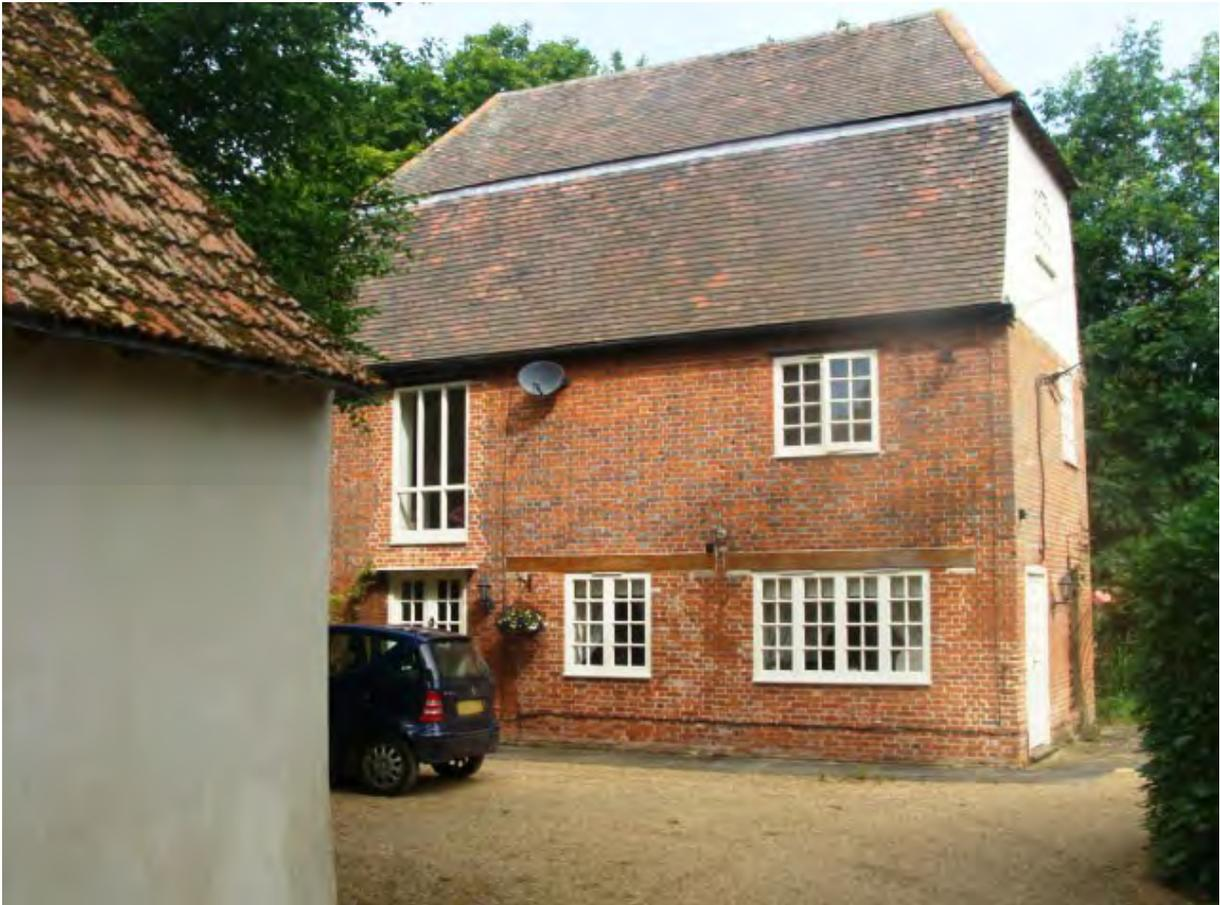
Picture 1.18 The Coach House to the west of Elmdonbury. Note wooden lintel interpreted as once having provided support for original entrance point.
