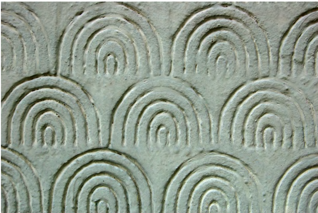
Picture 1.2 Traditional Essex combed pargetting of an unusual almost horseshoe shape on the wall of one of the Rickling Corner Cottages.
