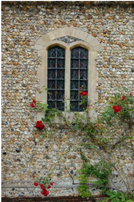
Picture 1.3 Local flint and imported stone contrast on the windows to the church of St Simon and St Jude, Quendon.
